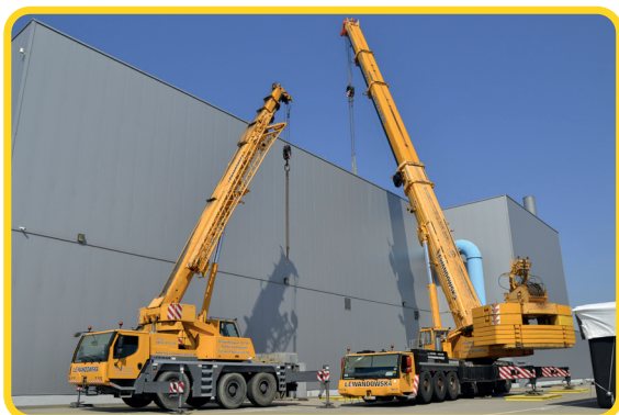
Cranes in action to replace the tank
